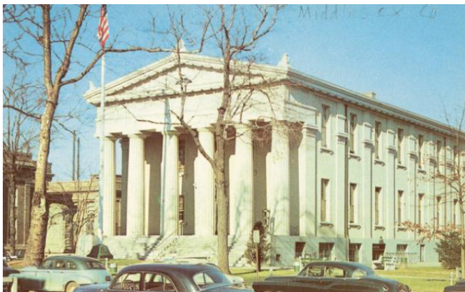
The old Middlesex County Courthouse, which occupied a block bordered by Bayard, Paterson and Kirkpatrick streets and Elm Row in New Brunswick.
