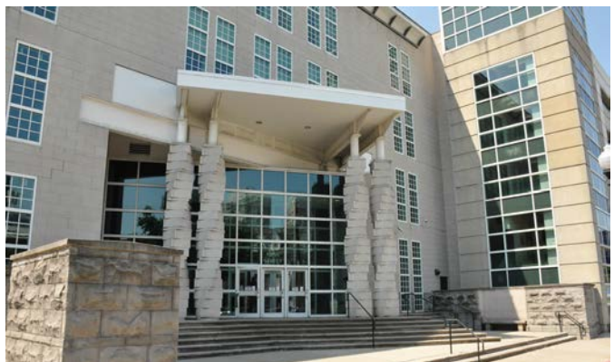
The Middlesex County Family Courthouse in New Brunswick as it appears today.
